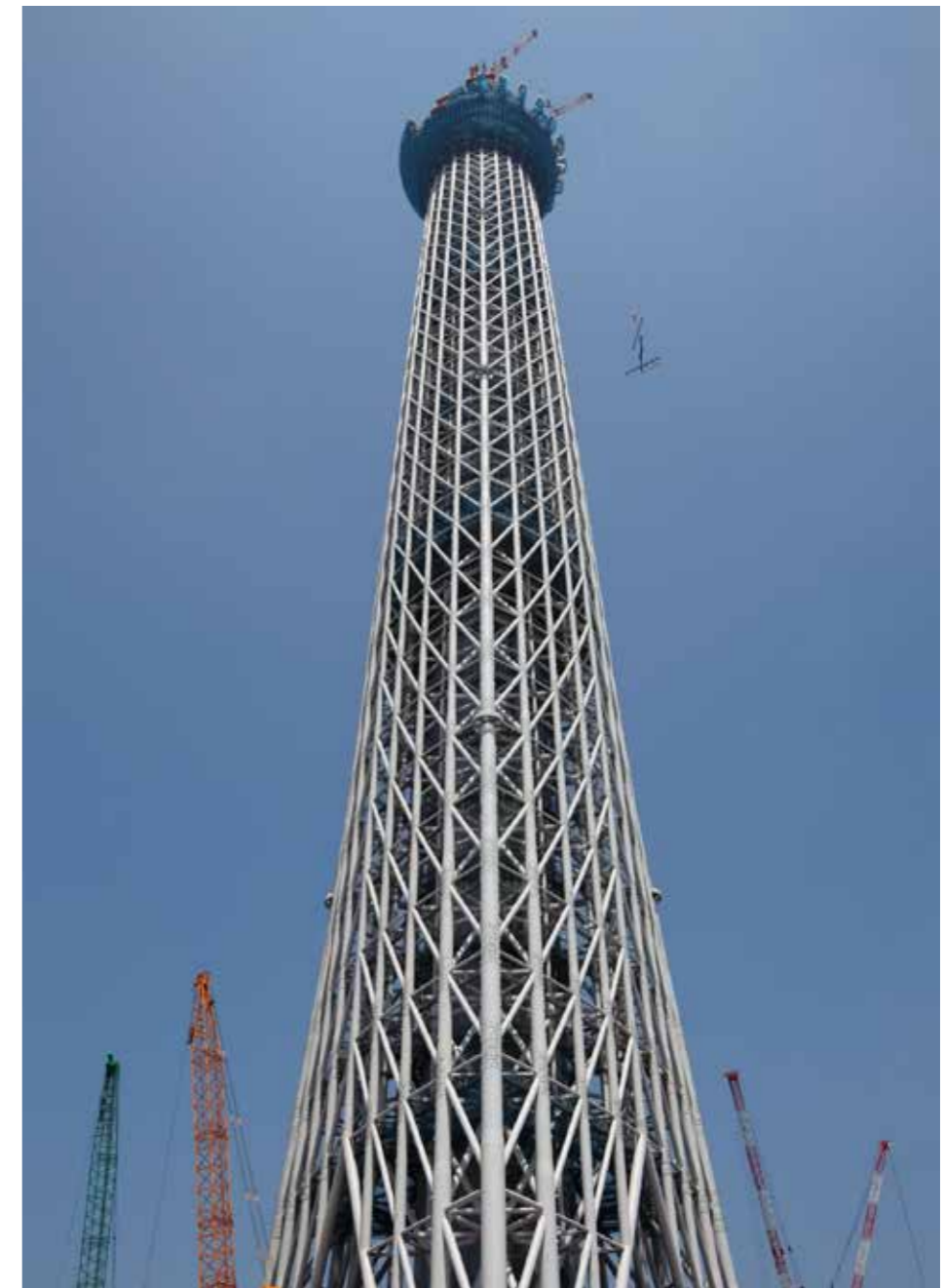
Sika's concrete superplasticizers were also applied in the highest broadcasting tower in the world: the Tokyo Sky Tree.
