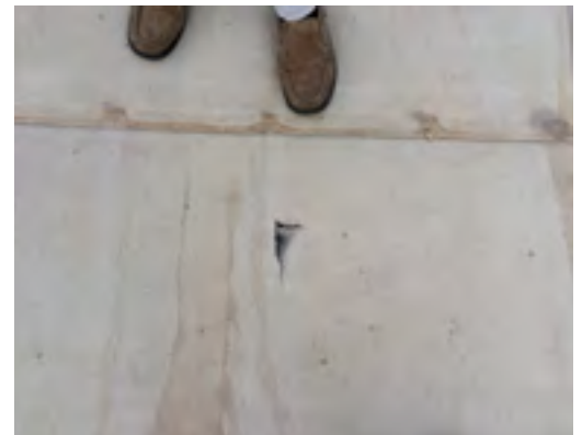
Cracks in the old roof.
