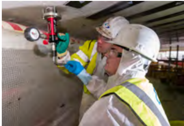
Pull-off test to test cohesive strength of concrete substrate after surface preparation
