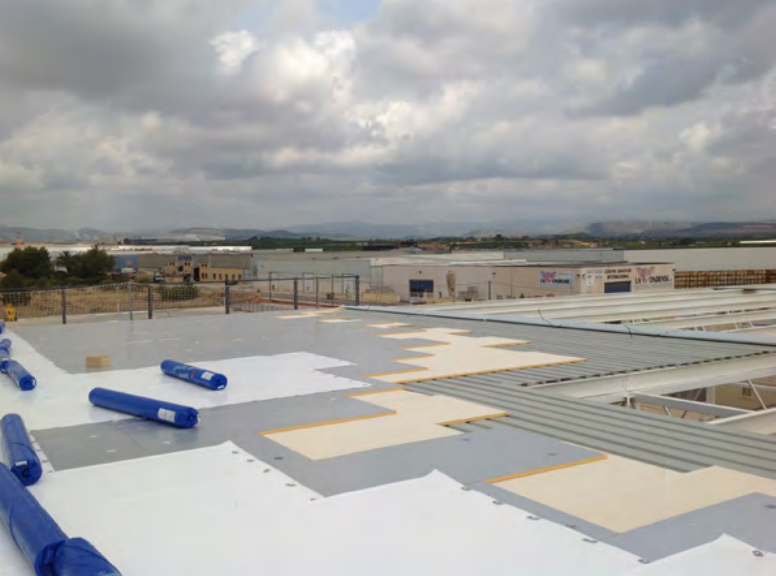
The results for a roofing system treated with beige Sarnafil TS 77-18 and one with white Sarnafil TS 77-18 SR demonstrate that both thermoplastic membranes bring significant savings.
