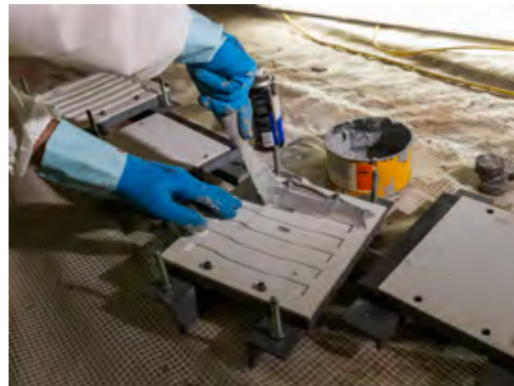
Application of Sikadur®-30 adhesive to carbon fibre plates.
