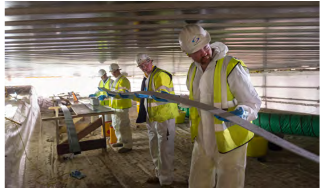
Installation of Sika® CarboDur® carbon fibre plates.
