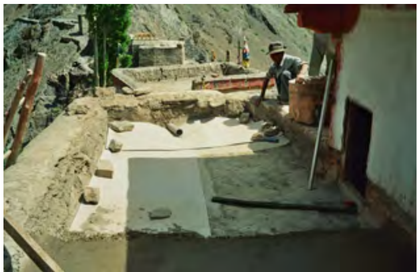
One particular problem during refurbishment was that the thickest – and thus heaviest – layer of the roof was resting on a relatively delicate ceiling structure, as evidenced by visible water damage inside.
