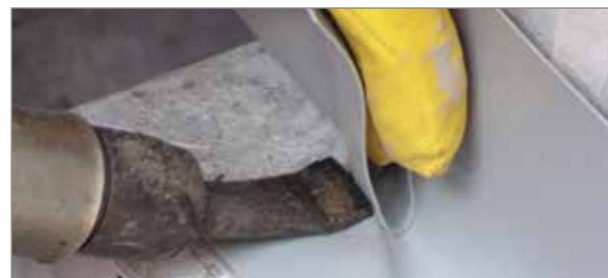
■ 4. Jointing membrane strips by heat welding
