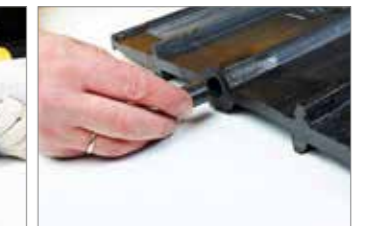
Plugging of the centre bulb with a cellular foam plug and inserting a raw rubber plug
