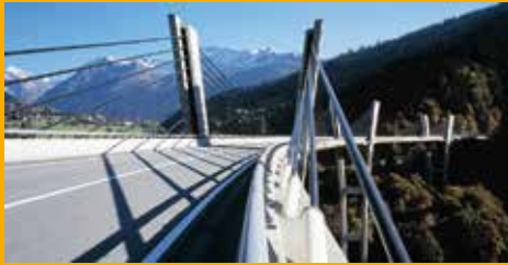
CONCRETE REPAIR AND PROTECTION
