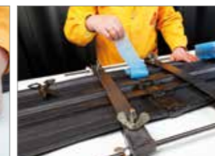
Jointing the waterstop, tightening with the fixing Clamps
