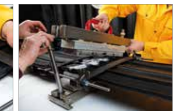
Powdering of waterstop and inserting into the vulcanizing equipment
