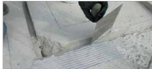
■ 2. Applying the base layer of adhesive
