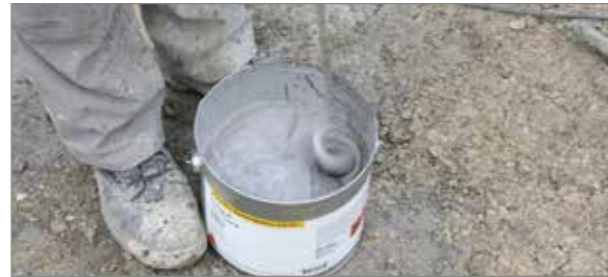
■ 1. Mixing the Sika® Tricoflex® FU 60 system adhesive
