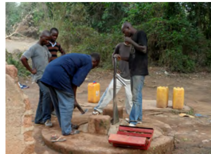
Access to clean and fresh groundwater has now been provided to the residents of 44 villages in total in Ivory Coast.
