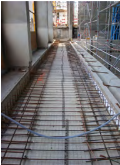
During works of refurbishment.
