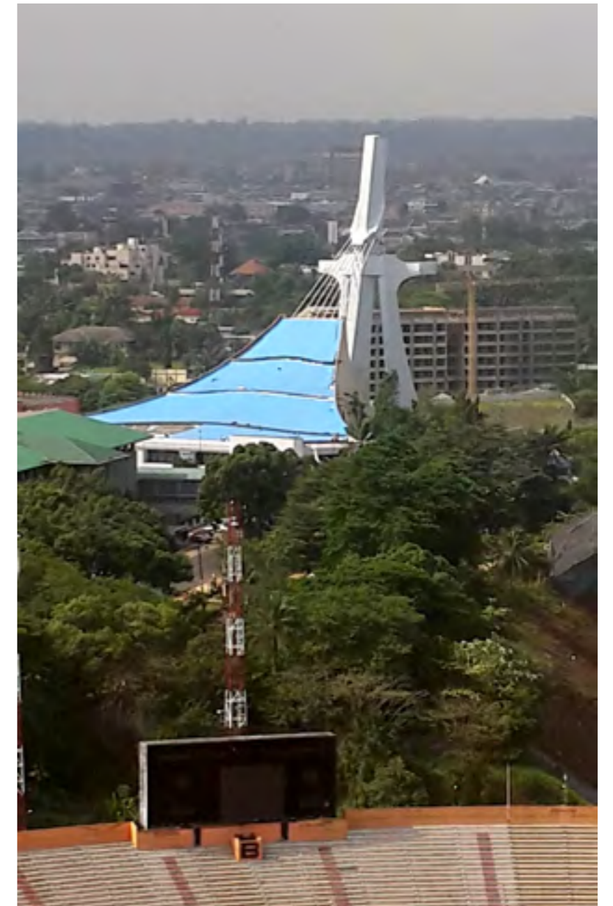
The roof of the Abidjan cathedral needed major refurbishment and Sika was chosen by the government to undertake this.
