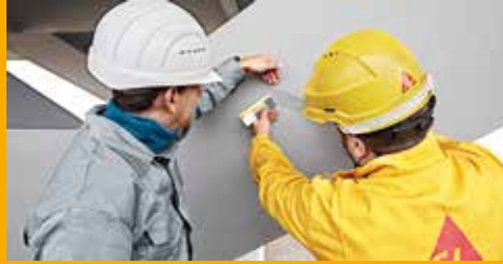
CORROSION AND FIRE PROTECTION
