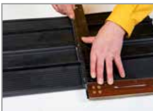
Measuring, marking, cutting
