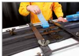
Joining the waterstop, tightening with the fixing Clamps
