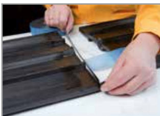
Applying the adhesion strip
