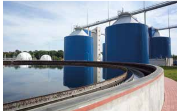
WASTE WATER FACILITIES
