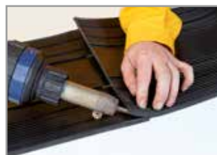
Overlapping joint with hotair blower
