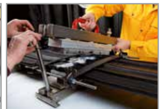
Powdering of waterstop and inserting into the vulcanizing equipment
