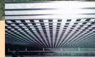
Applied CarboDur CFRP plates
