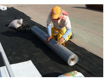
Construction in progress: placing protective geotextile over the concrete deck
