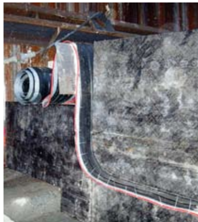
Back-up security for a water stop system
