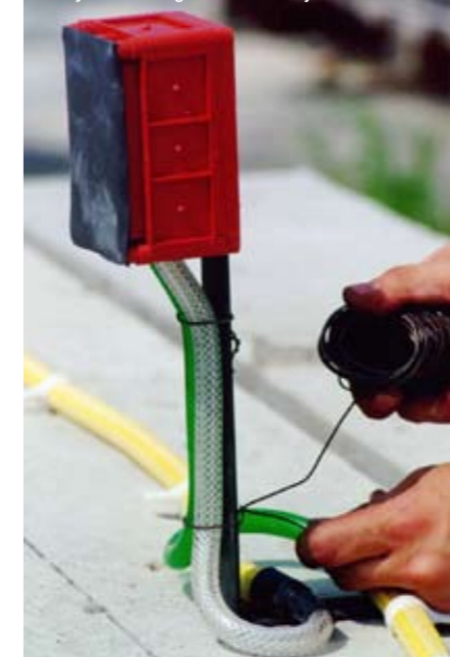
Easy connecting tool for the injection
