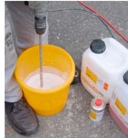
Mixing of an acrylic injection resin
