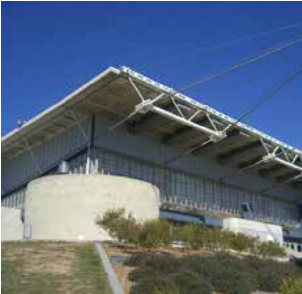
Project year: 1981 | Australian Institute of Sport AIS Arena Canberra, Australia
