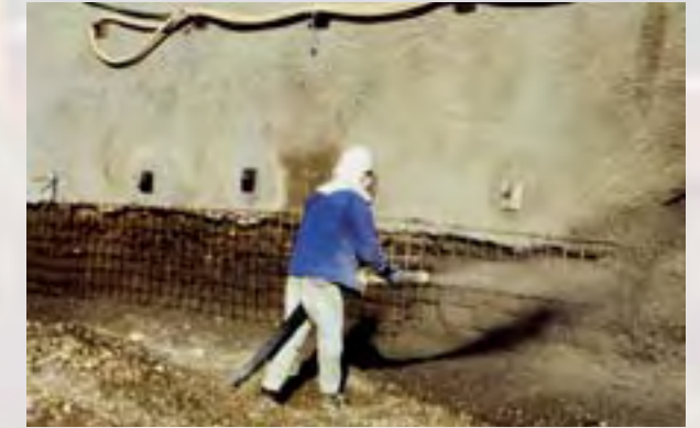
Excavation stabilization
