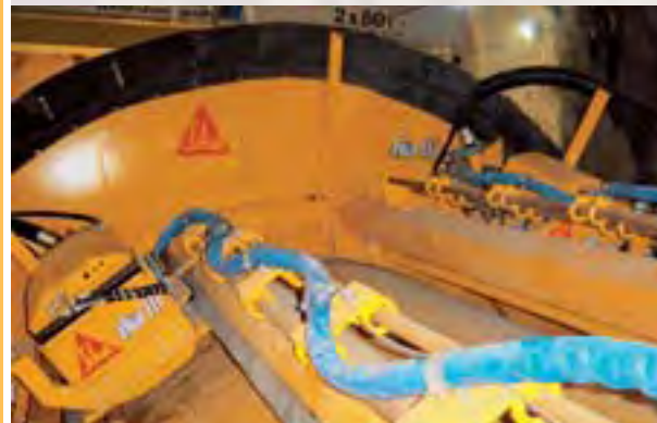
Shotcrete stabilization in TBM heading
