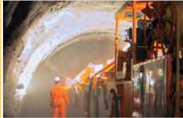
Sika-PM500 shotcreting system for large sections
