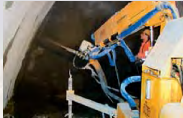
Aliva-503 shotcreting system for small sections
