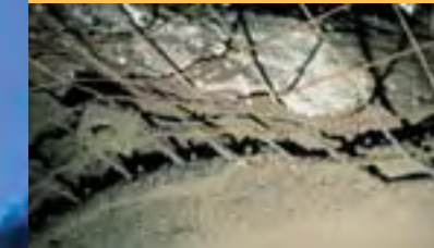
Concrete spraying, spraying shadow/rebound 2
