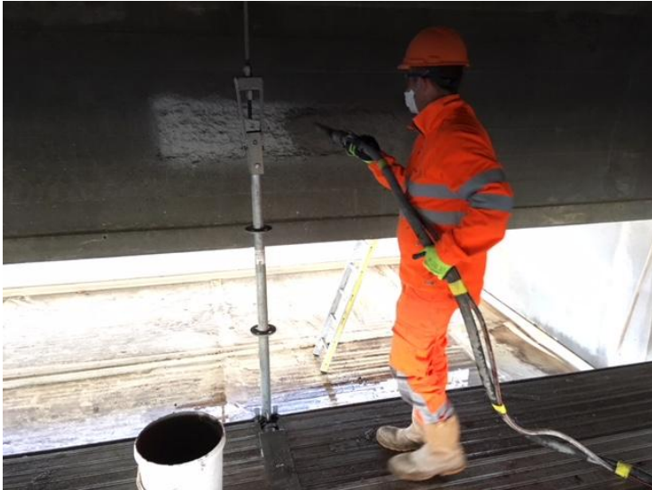
Figure 9. Spray application of Sika MonoTop®-4012
