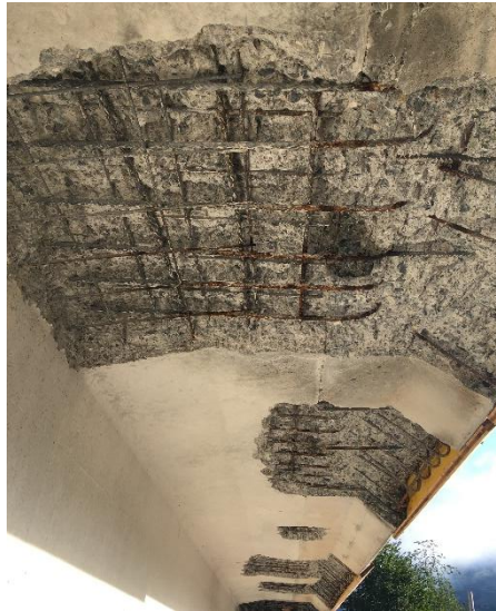
Figure 1. Substrate preparation by concrete removal with high water pressure and placing of formwork (right)
