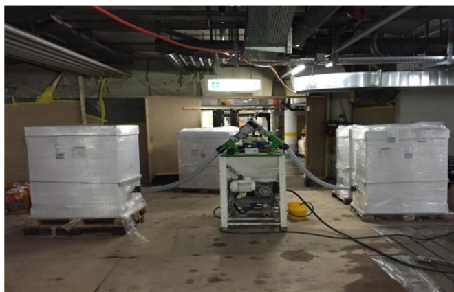
Figure 3. Inotec mixing pump with dust free material supply in one way containers (OWC)
