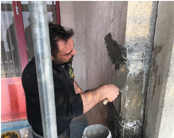
Figure 8. Hand application of repair mortar Sika MonoTop®-4012
