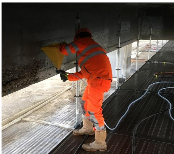
Figure 5. Application of bonding primer Sika MonoTop®-1010 with Hopper gun
