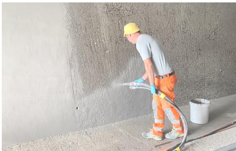
Figure 10. Application of Sika MonoTop-3020 by spray and hand application
