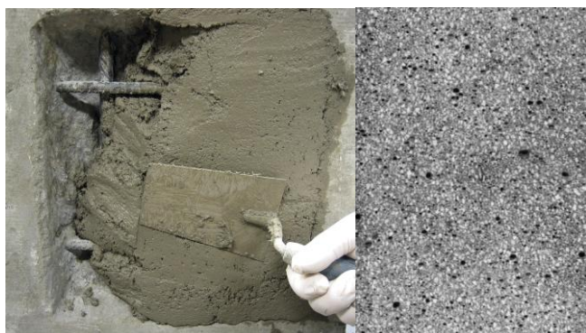
Figure 6. Hand applied mortar
