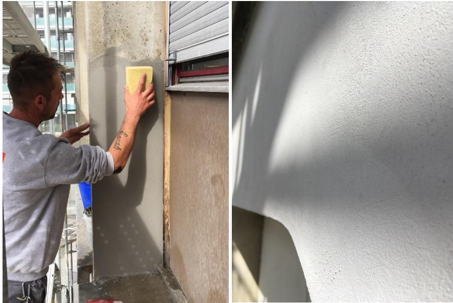
Figure 11. Finishing the levelling mortar Sika MonoTop®-3020 with a sponge
