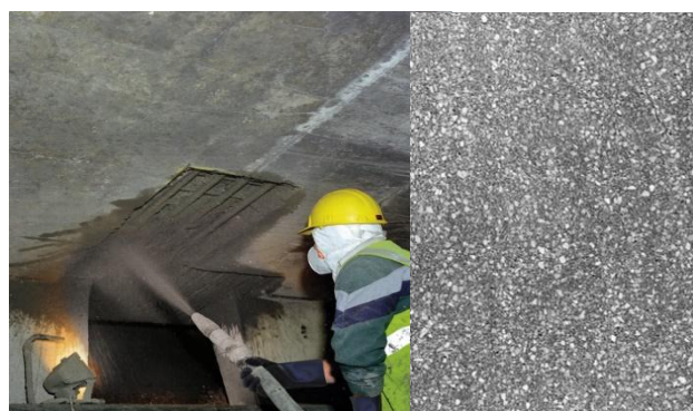
Figure 7 Machine applied mortar. More densely packed.
