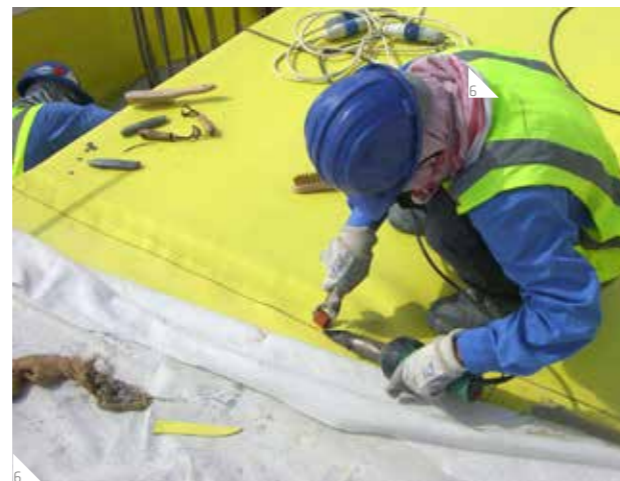
Compartmentalized sheet membrane systems
