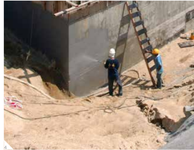
Liquid applied reactive membranes (PUR/PUA)
