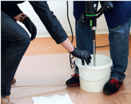
Manual mixing of 2-part Sikasil® GS 687 with cone agitator
