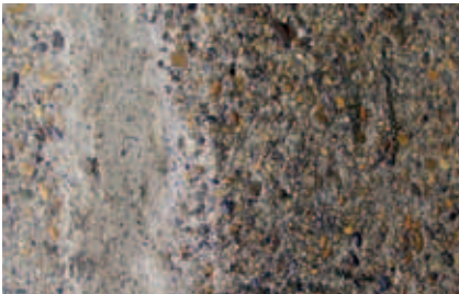
Fig. 8.7.5: Due to continuous exposure, the cement film is eroded in an initial step, and thereafter larger and larger aggregates are rubbed, knocked or washed out of the hardened cement paste.
