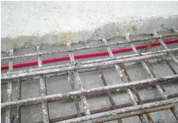
Construction joints
