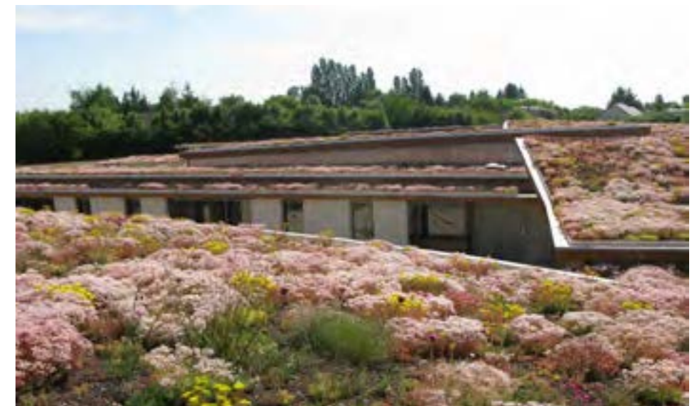
Project year: 2010 | Saint Douillard Medical Center, Cher, France Sarnafil® TG
