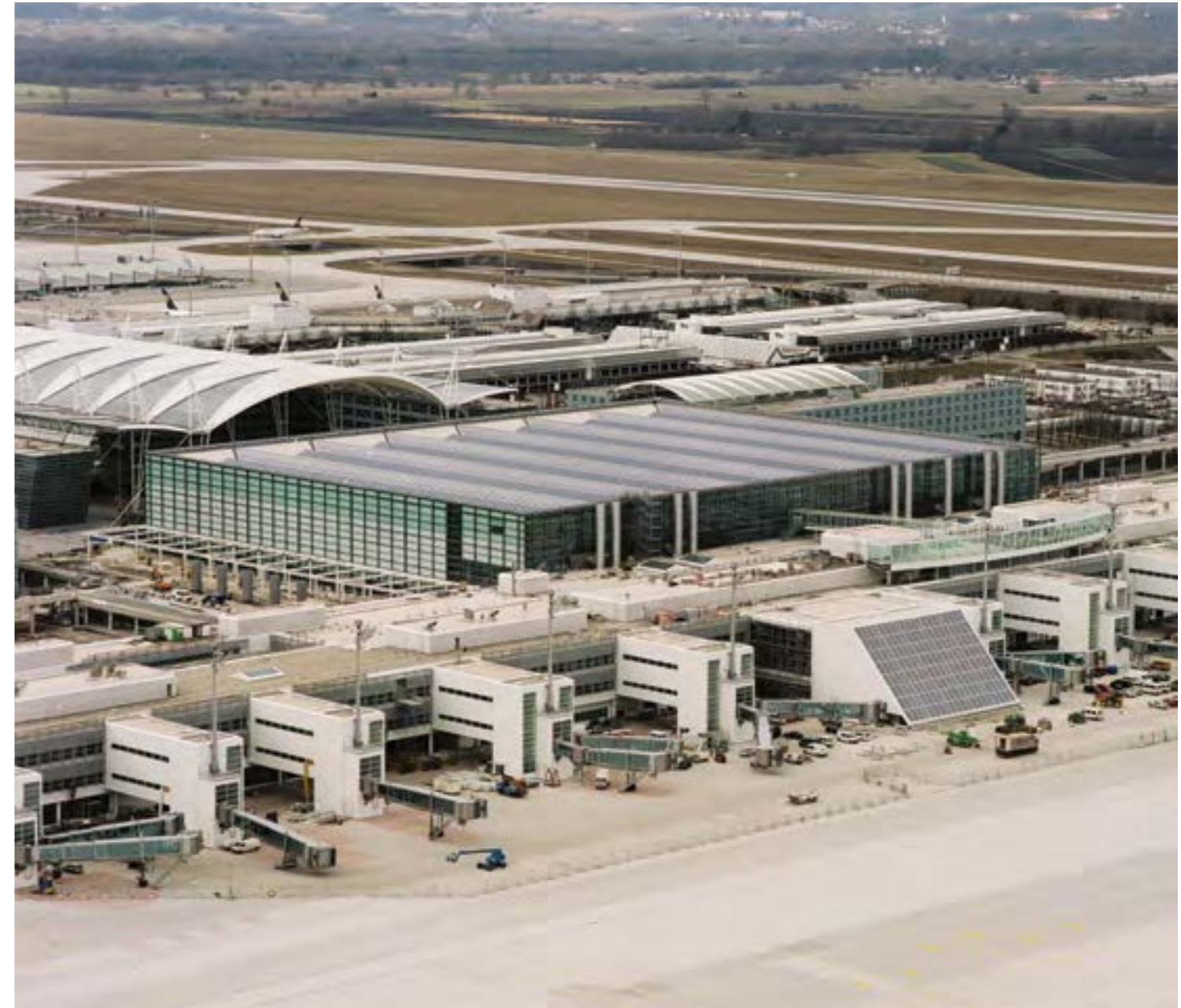
Project year: 1996 | Airport Terminal 2, Munich, Germany
