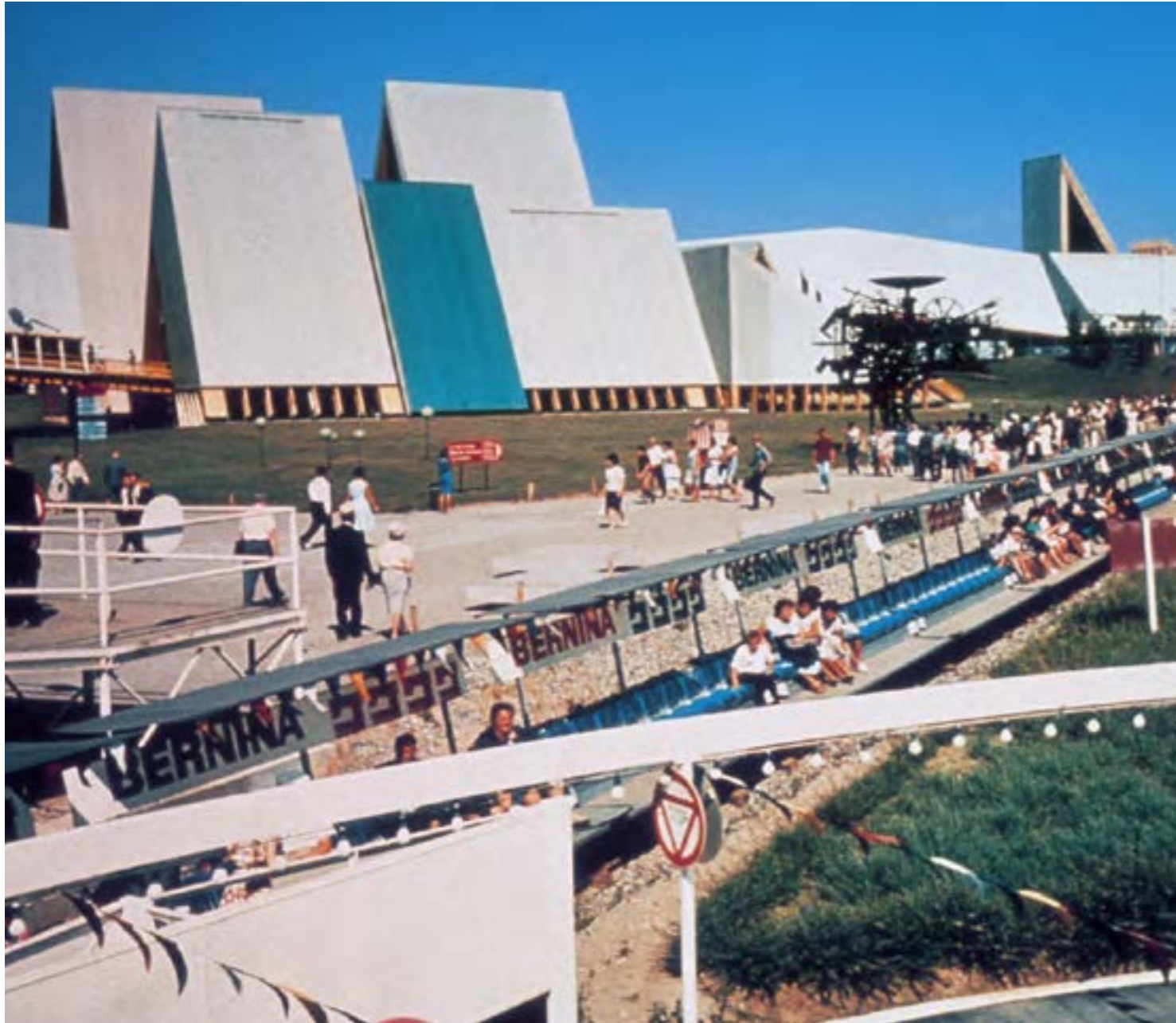
Project Expo 64 gave Sarnafil® the opportunity to waterproof a total of 42,000 m 2 roofs, including Swiss Path, Festival Hall, Military Pavilion and Monorail. This exposition introduced the Sarnafil® membrane to building professionals throughout the world.
