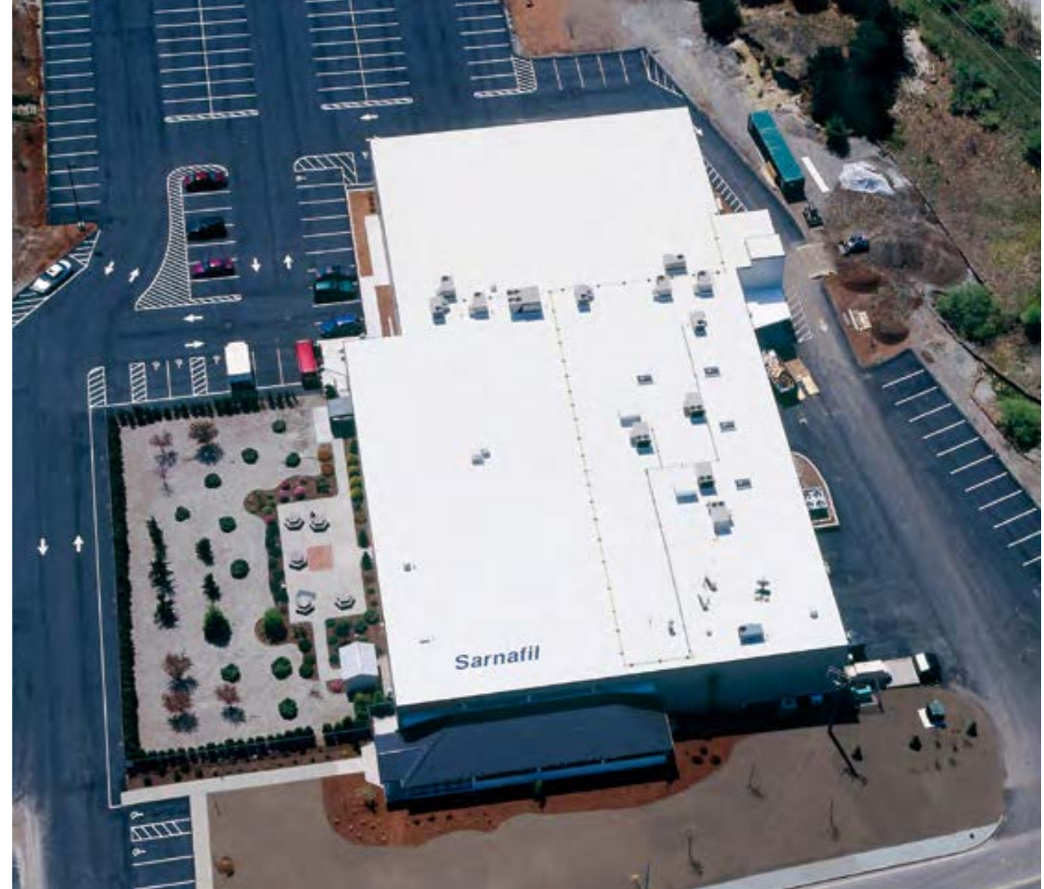
1998 | Introduction of EnergySmart white membrane to reduce building energy consumption due to its high reflectivity of sunlight
