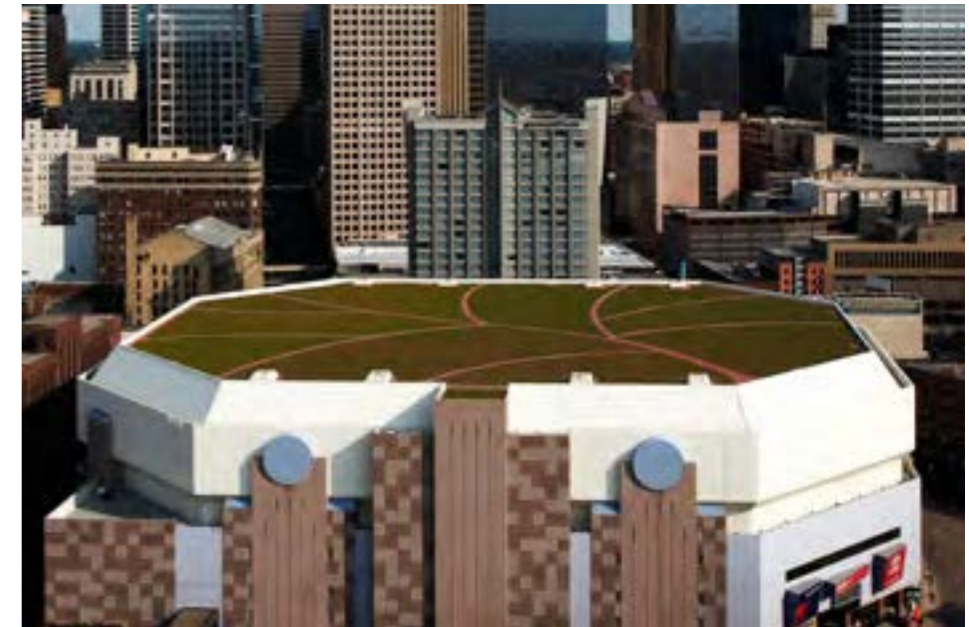
Project year: 2009 | Target Center Minneapolis, Minnesota, USA Sarnafil® G 476, Sarnafil® EnergySmart
