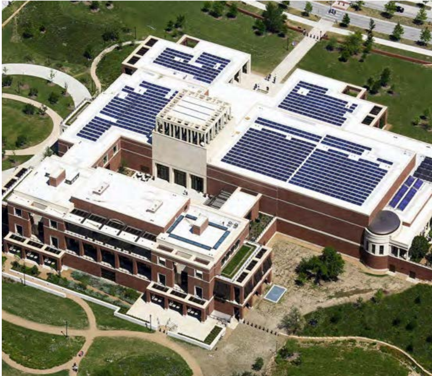
Project year: 2013 | George W. Bush Presidential Center, - Dallas, TX, USA Sarnafil® EnergySmart
