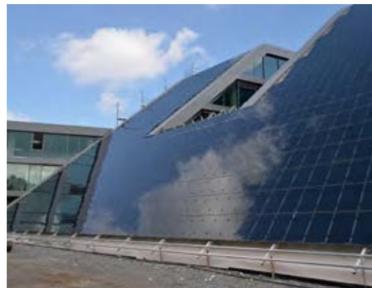
Project year: 2013 | Hahn und Kolb Administration and Logistic Center, Germany Sarnafil® TG 76 Felt, Sarnafil® TG 66 and SikaRoof® MTC 22
