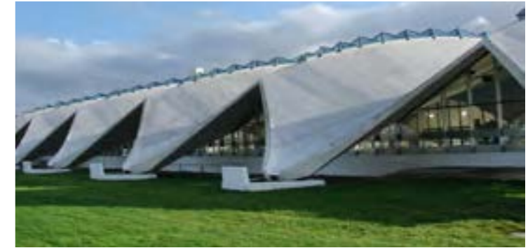
Project year: 1997 | Deauville Olympic Swimming Pool, Deauville, France | Sarnafil® T, white
