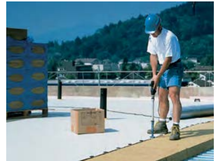
1979 | Mechanically fastened roofing system is introduced
