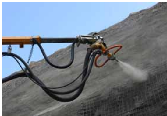
Fig. 2-3: Wet spraying
