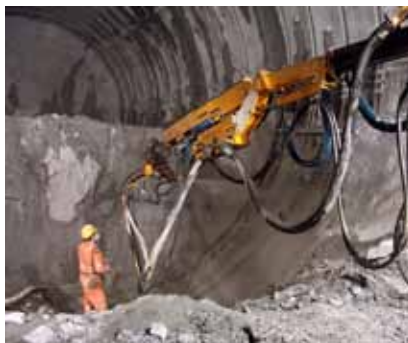
Fig. 3-9: Driving of crown method
