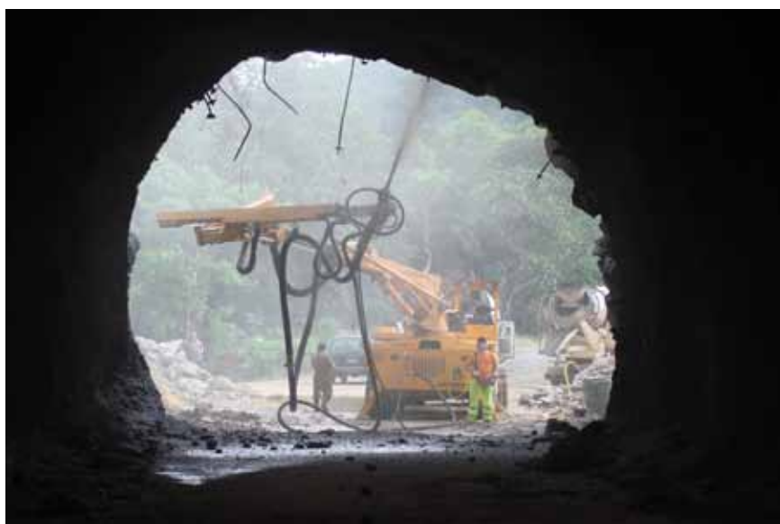
Fig. 2-1: Concrete spraying with Sika®-PM 500
