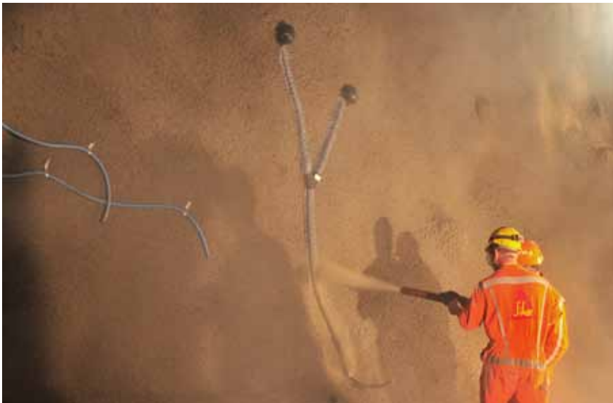
Fig. 11-3: Fixing of FlexoDrain W with Sika® Shot-3
