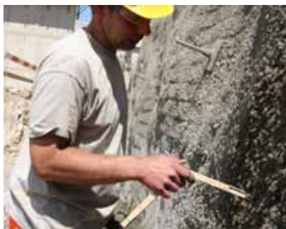
Fig. 8-13/14: Penetration of young sprayed concrete with studs using a Hilti DX 450-SCT (left) and measurement of the stud standoff for the determination of the penetration
