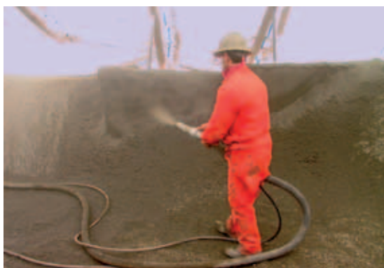
Fig. 2-2: Dry spraying
