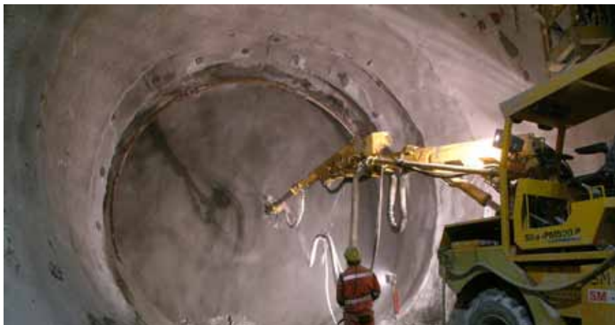
Fig. 3-1: Excavation stabilization with shotcrete
