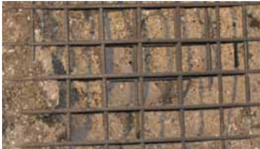
Fig. 5-6: High temperatures destroy unprotected concrete
