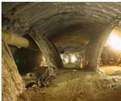
Fig. 3-8: Side wall method
