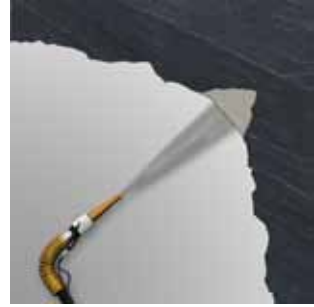
Fig. 8-2: Filling of overbreaks
