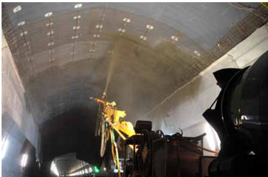
Fig. 3-10: Lining with sprayed concrete
