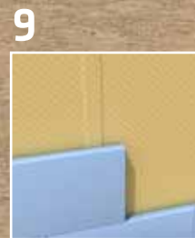
9 WT protection sheet/ felt and thermal insulation boards
