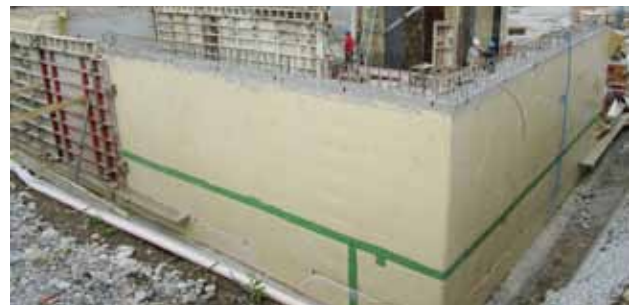
Open excavation with SikaProof® A, after removing the formwork the anchor penetrations has to be sealed.
