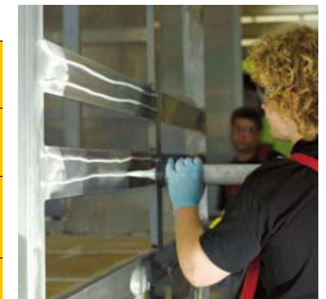
Bonding of the side wall on a aluminium structure
