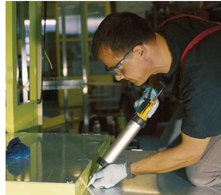
Sealing of the floor to the sidewall
