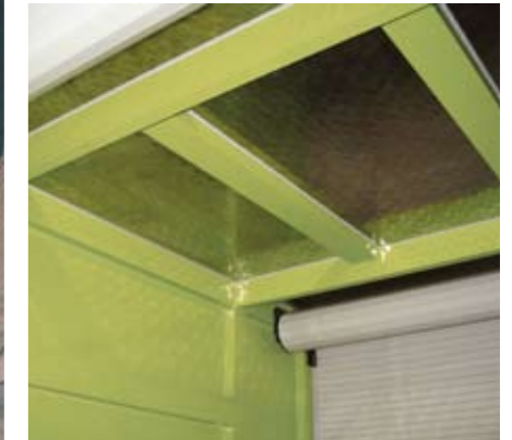
Sealed roof panel
