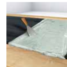
All steel cords have to be well embedded within the adhesive
