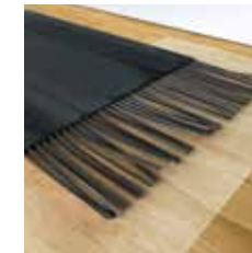
Prepare the belt to be jointed (Arrange the exposed steel cords)
