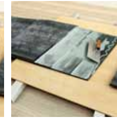
Evenly distribute the material to roughly 1 mm thickness
