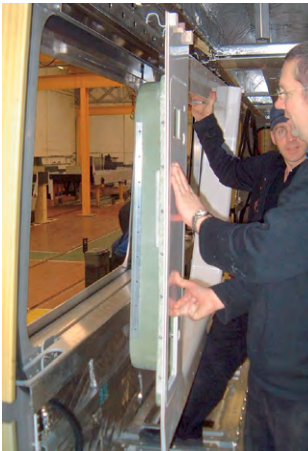
An interior panel is offered up prior to being fixed with Sikaflex®
