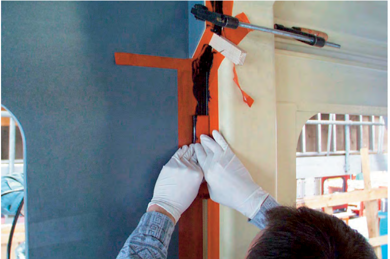
The joint between cab and main chassis, shown from the inside
