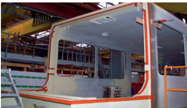
Various stages of construction using Sikaflex®
