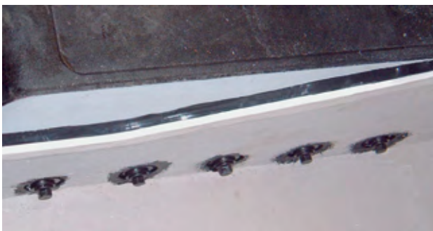
An interior joint is filled
