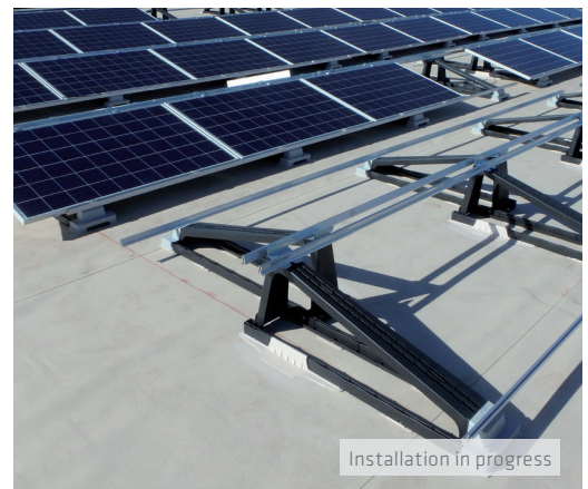
Hot-air welding of a Sika® SolarClick flange
