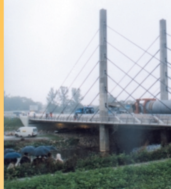
Heavy Truck Crossing the Bridge
