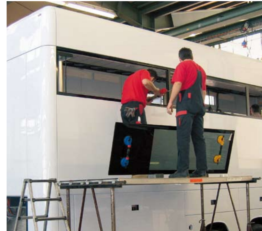
Direct Glazing with Sikaflex®
